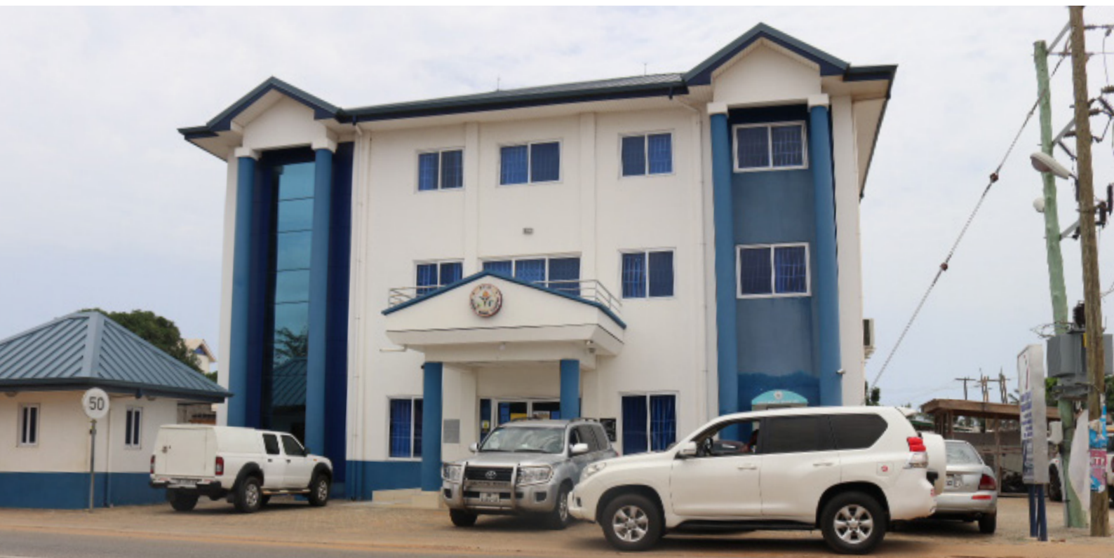
Head Office building of Anlo Rural Bank at Anloga
